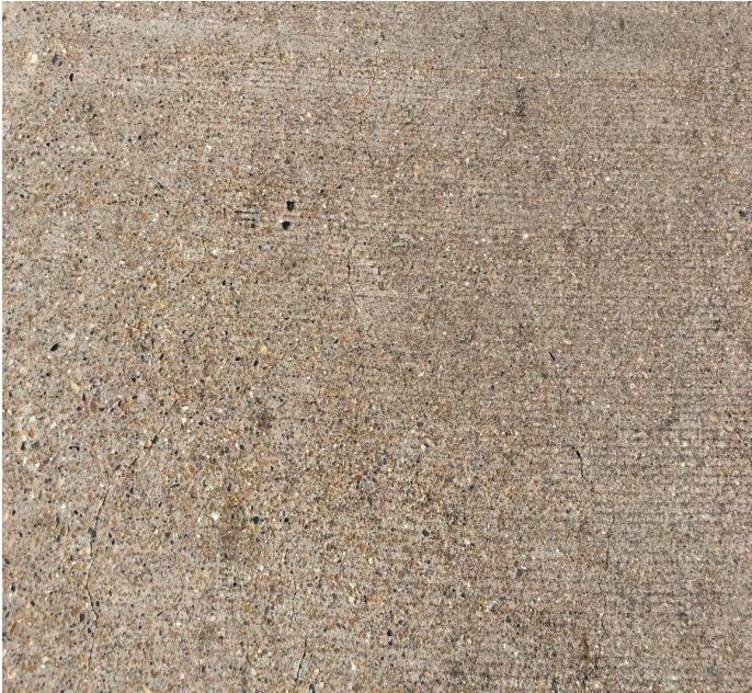
PHOTO 3 Description Deck map cracking
