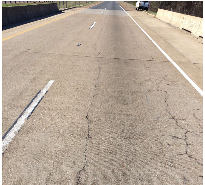
PHOTO 2 Description Cracks in deck
