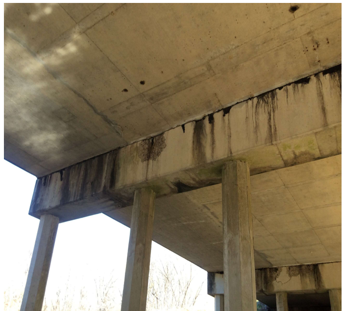
PHOTO 2 Description BT 17 spall 2 lf
