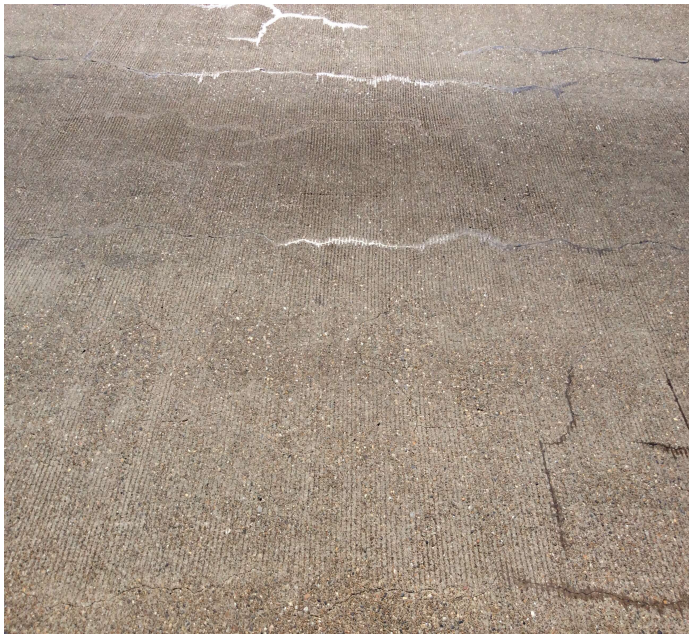
PHOTO 1 Description Cracks in deck some sealed some not
