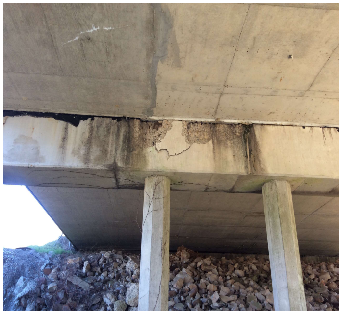
PHOTO 1 Description BT 18 spall on cap 6 lf
