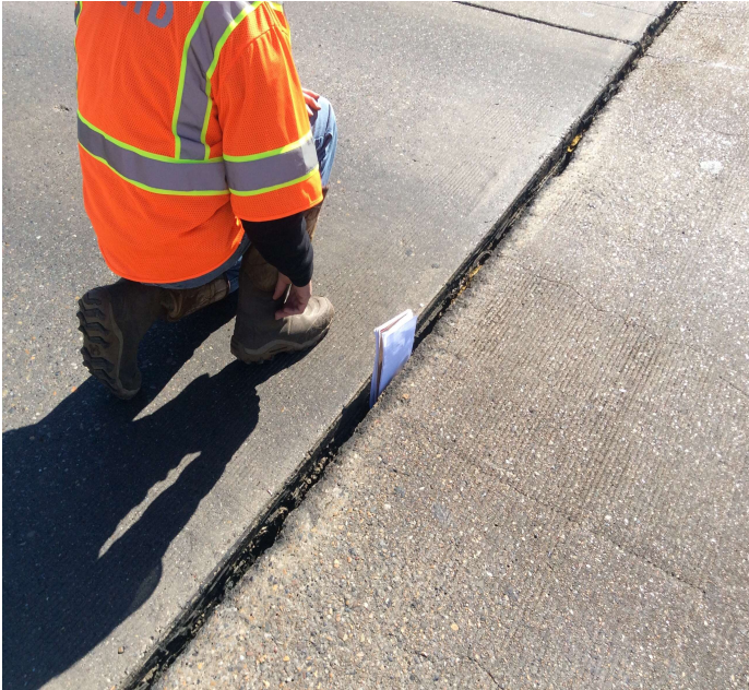
PHOTO 3 Description CONSTRUCTION JOINTS OVER BENTS JOINT MATERIA L IS COMING OUT OF JOINTS AT VARIOUS LOCATIONS.
